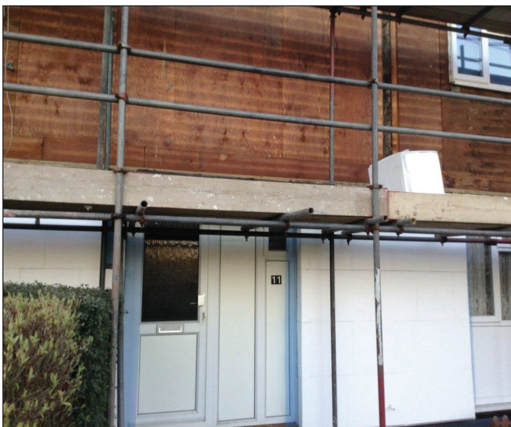
Retrofitting an existing house with external insulation
